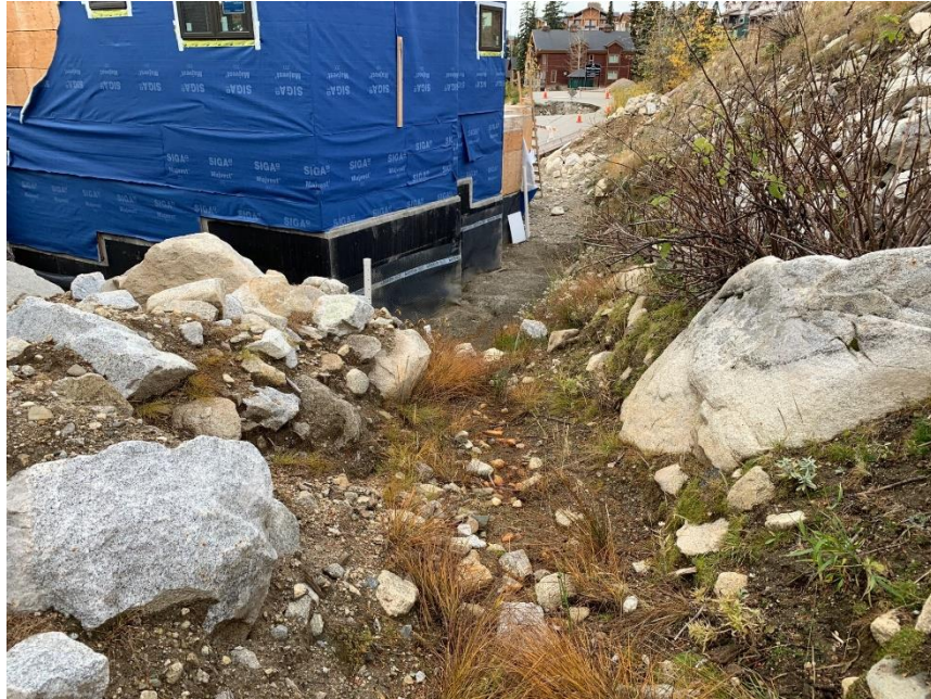
Figure 15 Existing drainage swale behind #2-200 Moonshine Cres. at toe of slope below Raven Ridge Road
