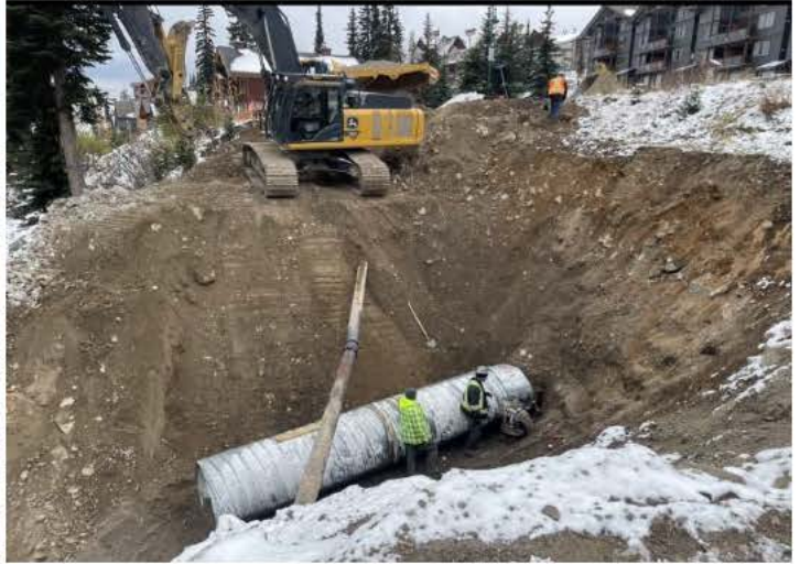
Water Main on top of culvert 15.9 feet.
