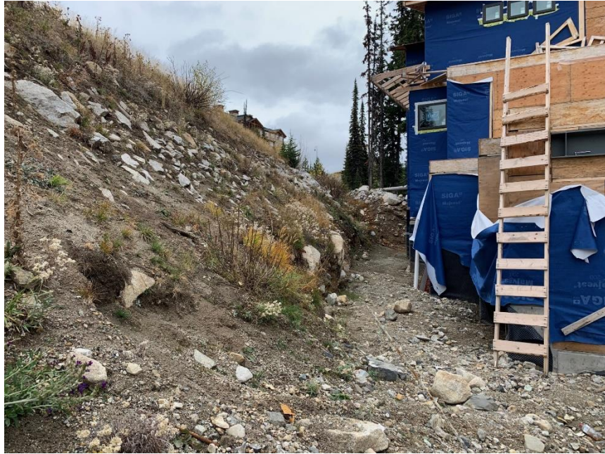
Figure 2 Slope Below Raven Ridge Road, Toe of slope has been excavated
