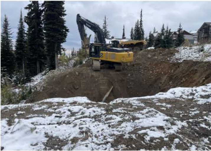
Entry to Bullet Creek: Water Main Exposed
